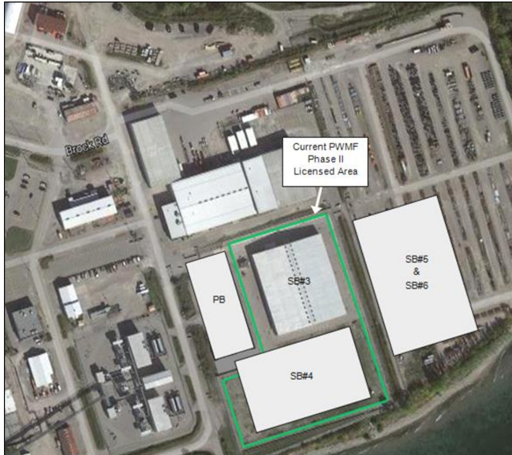
Aerial view of OPG's Pickering Waste Management Facility
